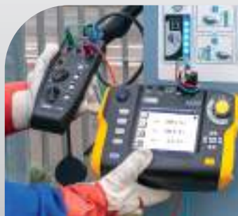
Monitoring of voltages delivered by a terminal with a 6 mA B/EV-type DDR during charging
